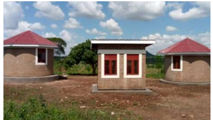
The completed teachers Tukulus at Victoria P/S
